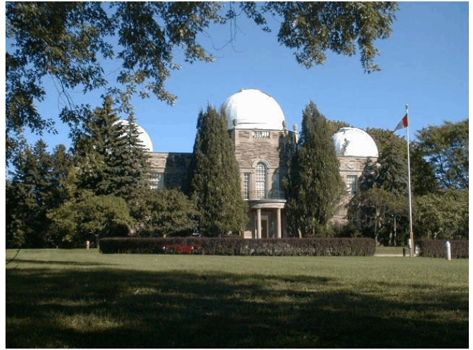
Figure 3 — The west administration building at the DDO.
