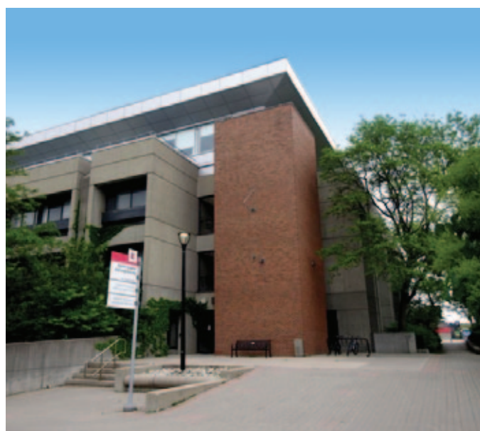
Figure 2 — R.M. Petrie Science and Engineering Building, York University, Toronto (Photo by DCM)
