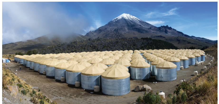
Figure 4 — The High-Altitude Water Cherenkov Gamma-Ray Observatory (HAWC) is a detector designed to look at gamma-ray emission coming from astronomical objects such as supernova remnants, quasars, and rotating dense stars called pulsars. Located roughly 4,115 metres above sea level near the Sierra Negra volcano in Mexico, the detector is composed of more than 300 tanks of water, each about 7.5 metres in diameter. Image credit: Jordan Goodman/University of Maryland.
