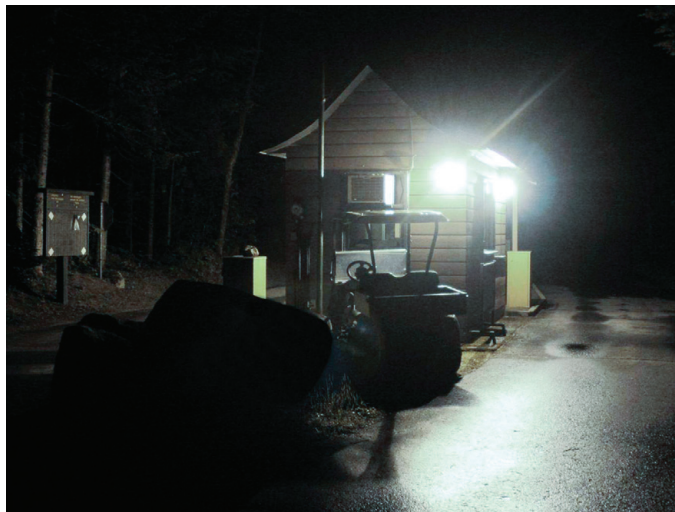
Figure 1 — The Entrance to a National Park. Unshielded wall packs shine into the eyes of motorists as they approach the kiosk. The luminance of the lamps overwhelms visibility in the area, and even the Stop sign. The glare masks any obstacles and hazards beyond the kiosk. The wall packs shine into bush and forest—disrupting the habitats and attracting predators and insects.
