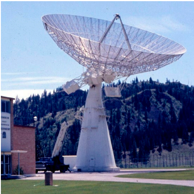
Fig. 1 — DRAO’s versatile John A. Galt 26-m telescope, commissioned in 1960 and in constant use ever since. Before the advent of the Synthesis Telescope, this was the observatory’s main instrument for cm-wavelength observations. At the atomic hydrogen \lambda 21 -cm line, it resolves angular detail of about half a degree.
