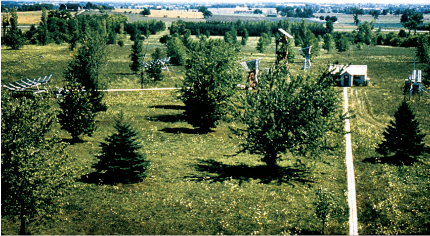
Figure 6 — Image of the DDO radio observatory, taken looking east from the roof of the DDO Administration Building, ca. 1960. The two antennas on an east-west baseline to the left are wire mesh parabolic cylinders used together with one of the pyramidal horns in an early phase of the interferometric work on discrete sources. At centre right are the two pyramidal horns arranged as an east-west interferometer and used in the final phase of this work. They are shown straddling the mounting tower for an unrelated “zig-zag” antenna used for solar measurements. The radio shack housing the receiver is clearly visible. The antenna to the immediate right (south) of the radio shack is a prototype segment of an east-west array intended to be part of a much longer array at 707 MHz at the Algonquin Radio Observatory. This array was never built, and the prototype section was never used as a radio telescope on its own (reproduced courtesy of the Department of Astronomy & Astrophysics, University of Toronto).
