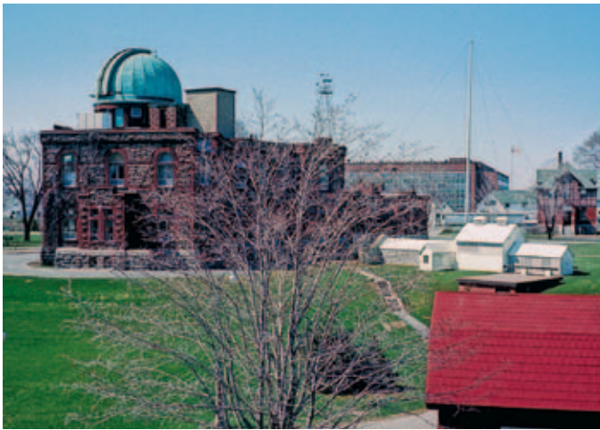
Figure 3 — The Dominion Observatory viewed from the NE in April 1967. The white structure houses the mirrors that comprise the horizontal solar telescope.
