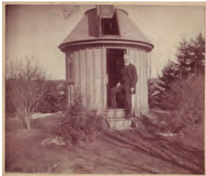
Figure 2 — John Goldie outside his observatory in Galt. His equatorially mounted refractor is visible through the open door and dome. The structure is typical of small 19th-century observatories, although the woodwork and finish appear to be quite superior. The design, known as the “Romsey Observatory,” is the Victorian equivalent of the SkyShed POD. It was developed by the Rev’d Edward Lyon Berthon (1813-1899), and was meant to be a solid, adaptable, low-cost alternative to other structures. The design would probably work as well today as in the days of Queen Victoria (Berthon 1864). The Romsey Observatory would have been a familiar sight on the 19th- and early 20th-century Canadian astronomical landscape; have any survived?
