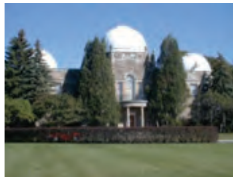
Figure 1— The western side of the administration building, the best-known view of the observatory. Image courtesy Slavek Rucinski.
