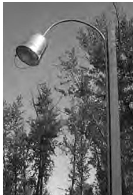
Light bucket — a whimsical, ready-made light shield in Winthrop, WA, photograph by Bruce Weertman of Dark Skies Northwest. Is the owner an astronomer per chance or was a bucket the first thing in hand in this rural community south of the Okanagan?
