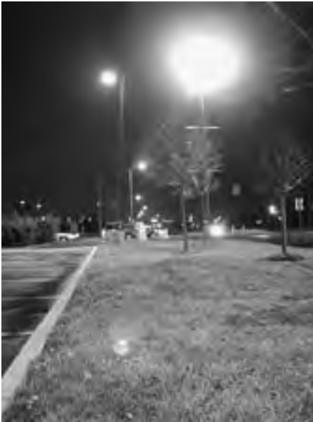
Scott Griswold's photo of a full cutoff (FCO) light fixture and a drop lens 'glare bomb' gives a good comparison of their different effects but is not the same as the human eye perceives.
