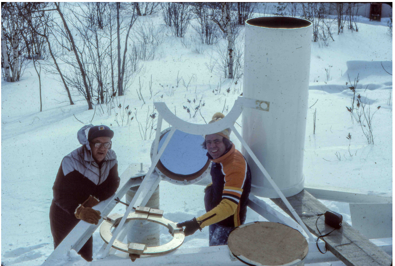
36 - 853 (February 1985, Top) Steve and Ken Odaisky prepare to install the Primary Mirror. 37 - 854 (Bottom) Ken and Steve moments after Primary Mirror Installation. The White tube will enclose the Mirror and Protect it, while allowing passage of the focused beam of Sunlight up the Polar Axis.
