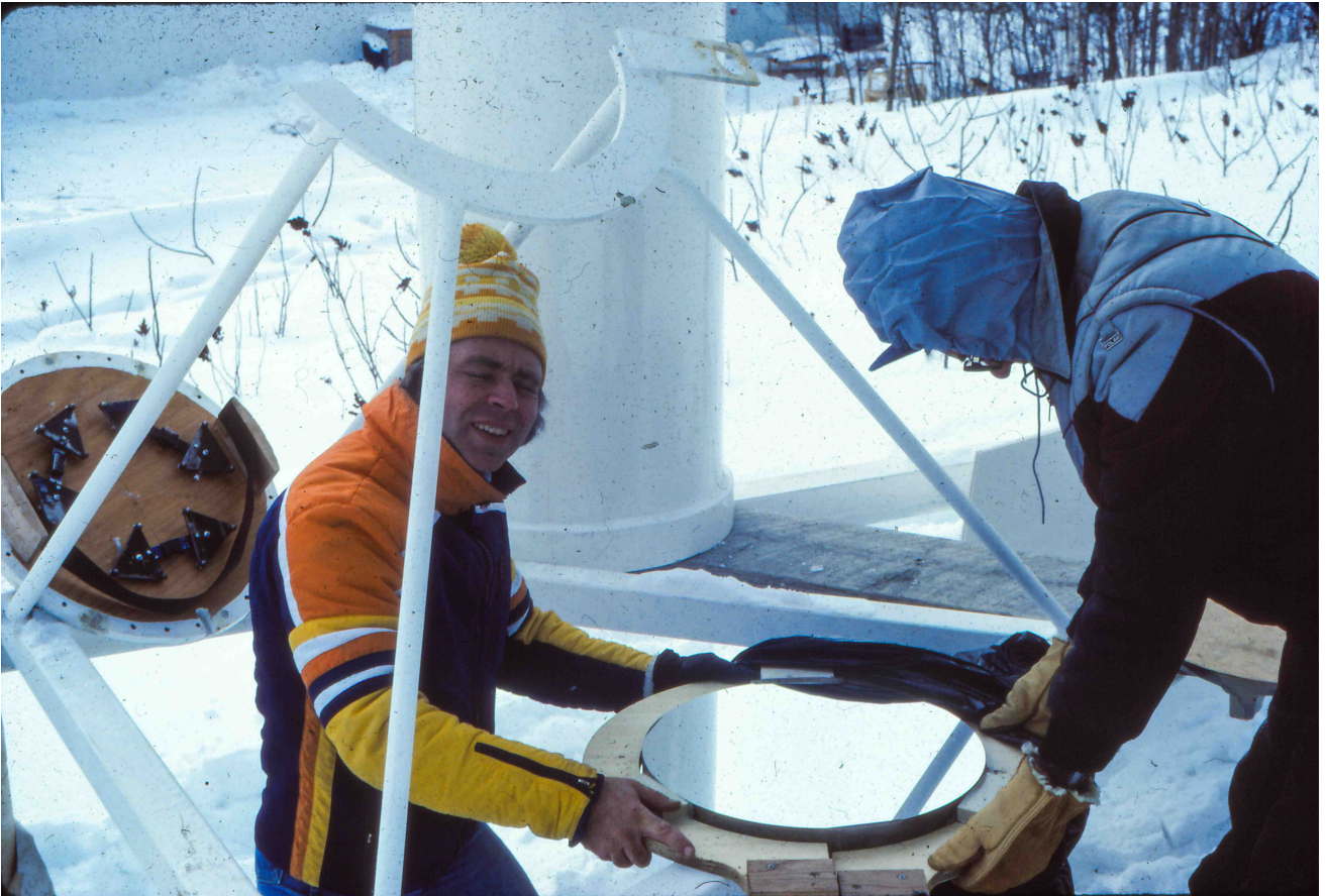
36 - 853 (February 1985, Top) Steve and Ken Odaisky prepare to install the Primary Mirror. 37 - 854 (Bottom) Ken and Steve moments after Primary Mirror Installation. The White tube will enclose the Mirror and Protect it, while allowing passage of the focused beam of Sunlight up the Polar Axis.
