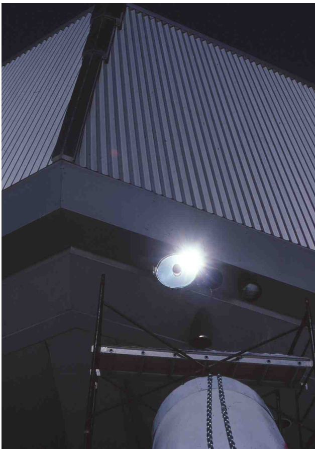
18 - 896 (left): The Beam Tubes are hidden in the glare of sunlight reflected off the perforated Flat Mirror downwards to the imaging mirror in the white tube. (right) 19 - 897: The result is focussed beams of sunlight inside the Observatory. (Both photos from March 1985)
