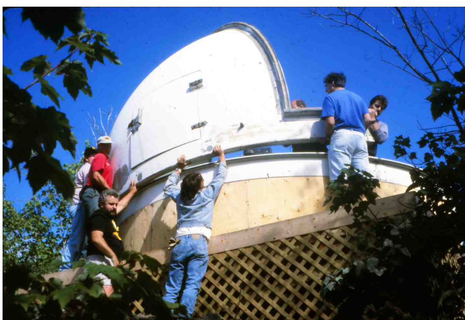
(47 - 1908, Below) Locating the Dome Half on it's Track)
