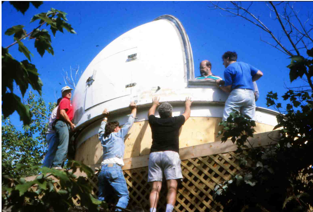
(48 - 1909, Saturday August 28/1993) Engaging the First Dome Half on its Track. Greg Beach (Black Shirt) and Alan Ward (Blue Shirt) lifting. Bob Ulrichsen is inside the Dome guiding.
