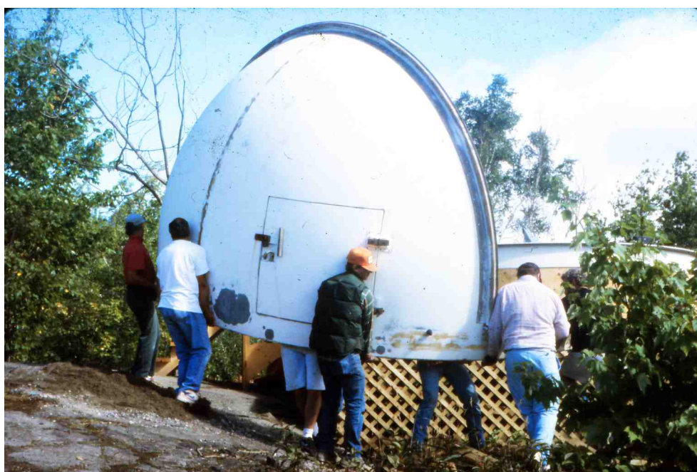
(46 - 1904 Lower Left) Lifting the Dome Half into Place.
