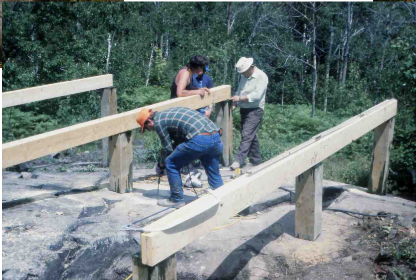
(39 - 1879) Dennis drilling into the rock to install post- securing hardware (Left)
