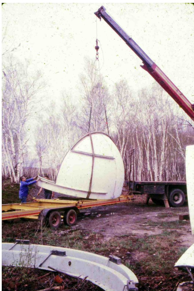
(25 - 1834) Crane Lowering the Dome Half onto the Trailer - Dome Track in the Foreground
