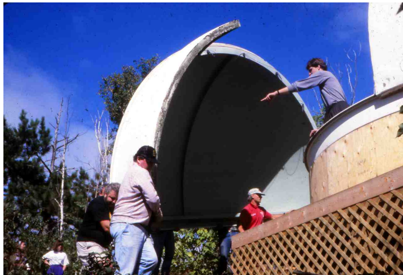
(52 - 1920, Above, Middle Left): Preparing to Lift the 2nd Dome Half
